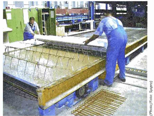
Fig. 1 Production of thermal walls in the precast concrete plant: inserting the insulation layer.
